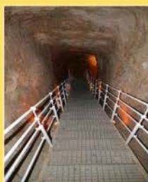
The inhabitants of the Canaanite city used this secret tunnel to descend from the city level (667 m high) to the spring level (635 m), to fetch water
